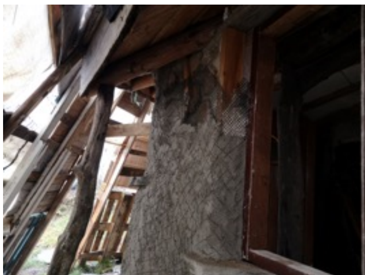
12. Attaching & plastering oyster bags
