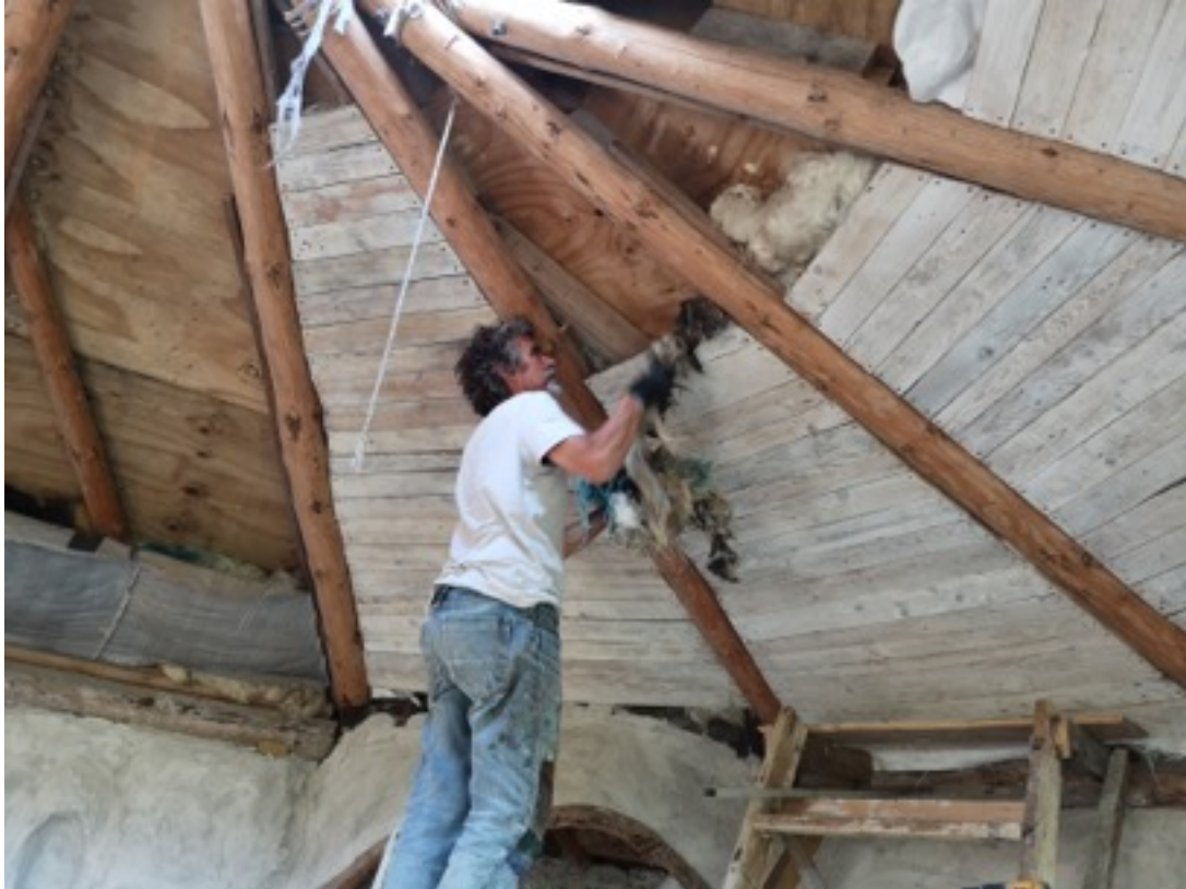
7. Wool insulation on ceiling
