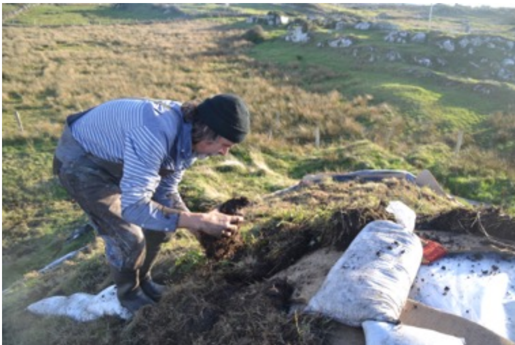
11. Placing turf back on roof
